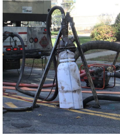
CIPP Liner Installation
