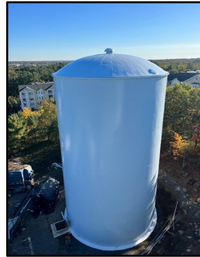
Rehabilitated Water Storage Tank
