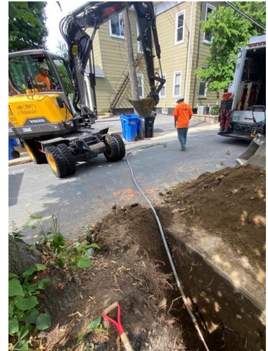
Lead Service Line Replacement
