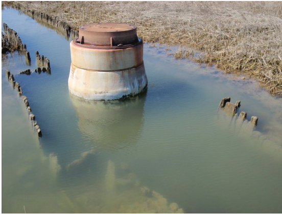
Sewer Manhole in Marsh: Raised and Sealed
