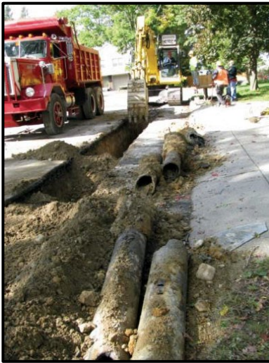
Water Main Replacement Construction
